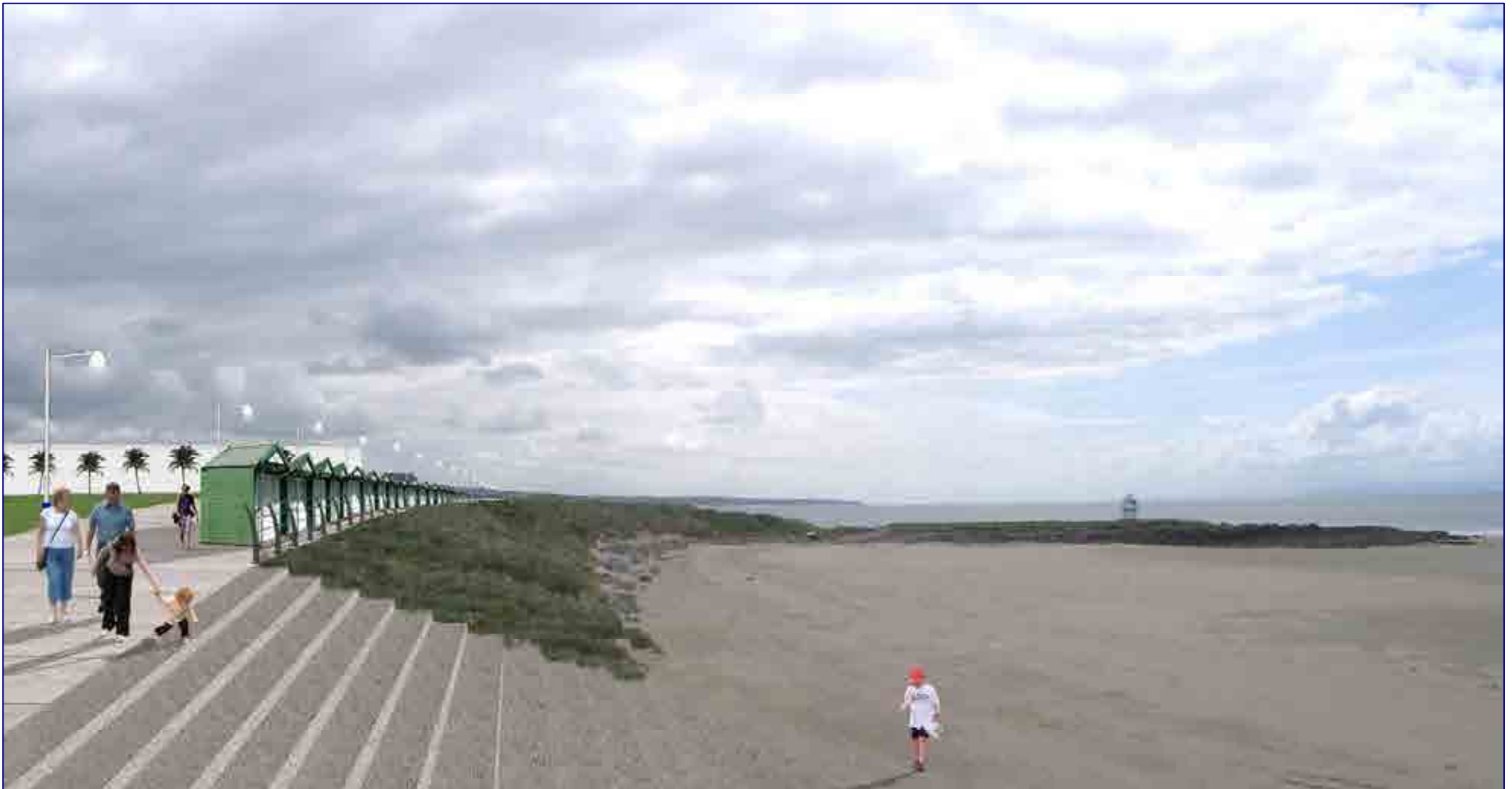
Photomontage 6 - Artist's impression of the promenade and sea defences in front of Foreshore Park, showing the transition between the stepped revetment and rock revetment.
