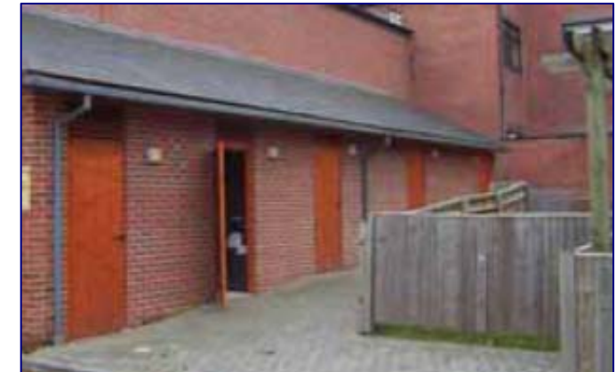
Examples of effective bin storage.
