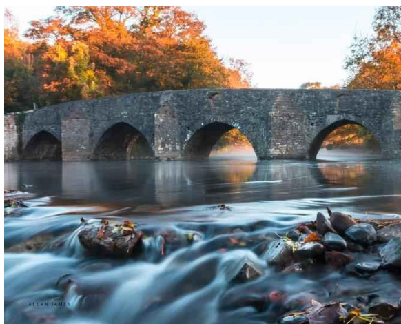
New Bridge, Merthyr Mawr, Bridgend
