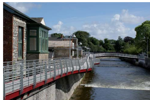
③ From 'Old Bridge' towards new cantilevered boardwalk
