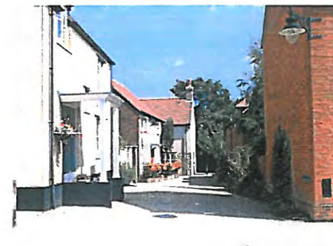
Street furniture is carefully designed to complement the character of the development. The obtrusive clutter of street signage and furniture is minimised, as here, where lighting is positioned on the building.
